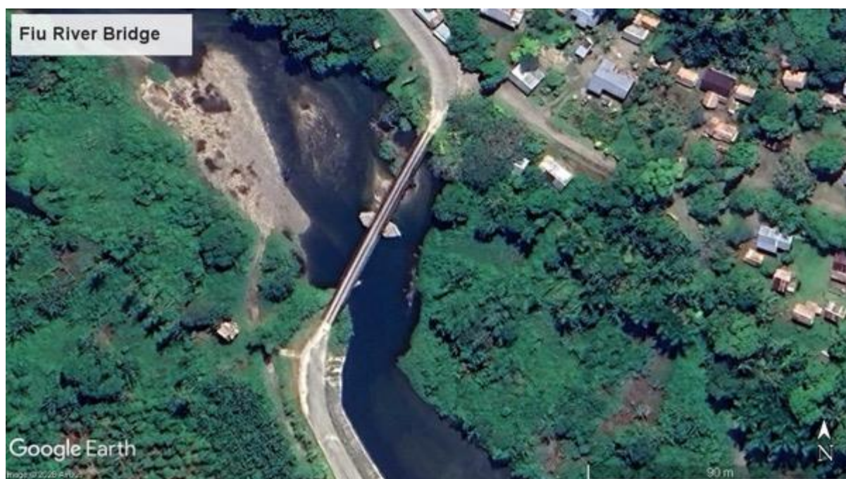
Figure 1: Fiu River bridge
