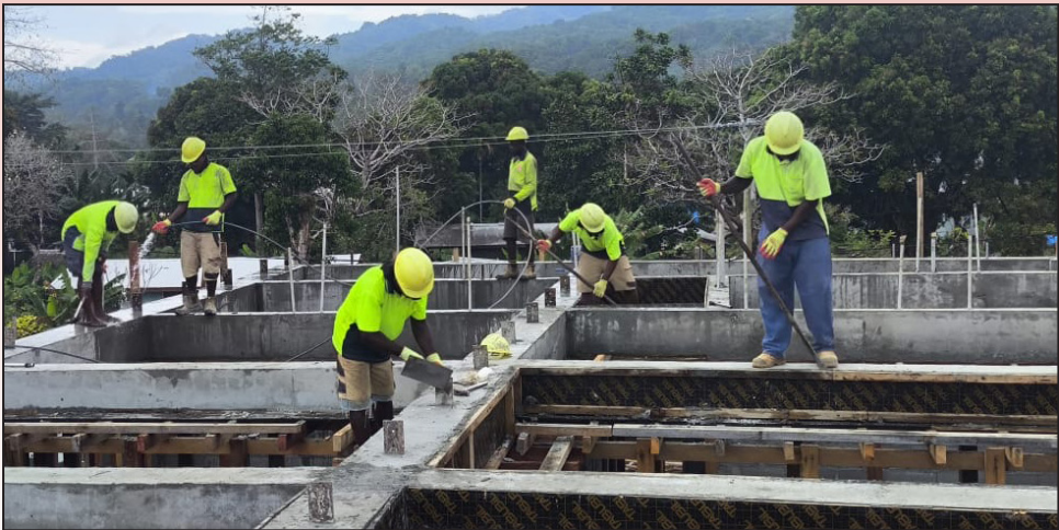
Construction of MALD Extension Office Building Kirakira, Makira Ulawa Province
