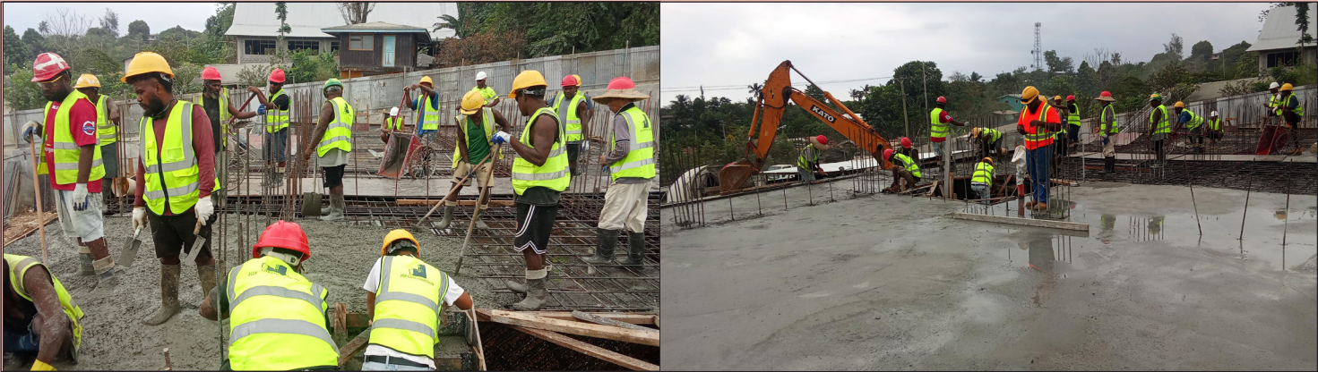
Construction of the MALD Extension Office Building in Auki Malaita Province
