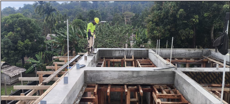
Construction of MALD Extension Office Building Kirakira, Makira Ulawa Province
