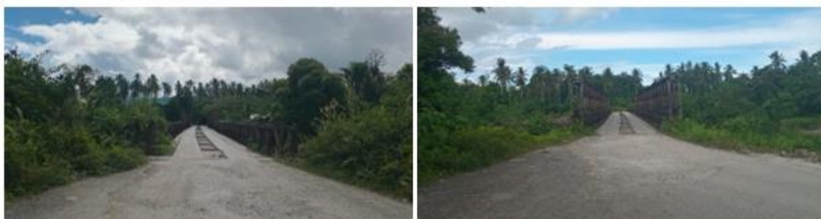
Figure 6: Fiu bridge view from the Southern and northern approach
