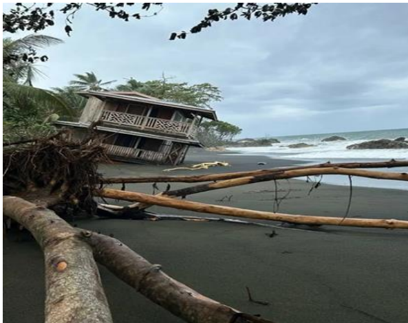
Dwelling house damaged, photo source: Ileen Zama
