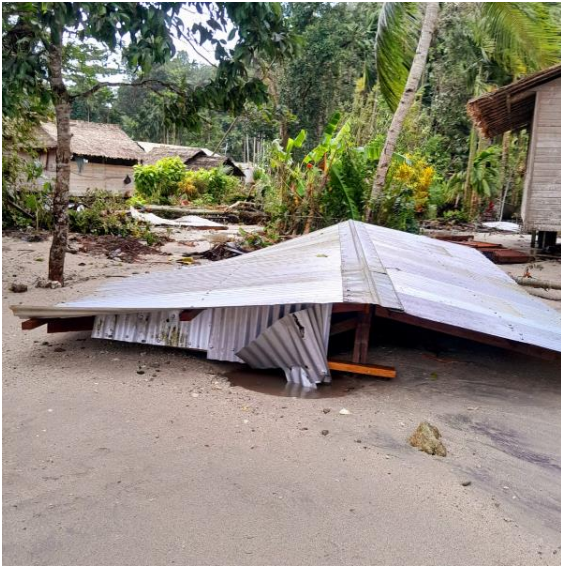
Dwelling house destroyed in Leona Village, North Vella la Vella. Source: +6777481932
