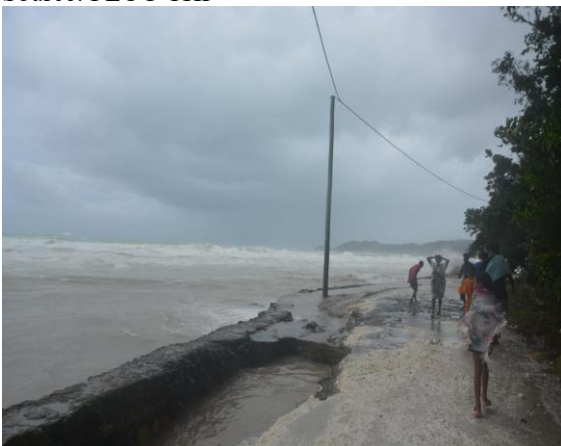
Destruction to roads, Titiana Village, Gizo. Source: PEOC WP
