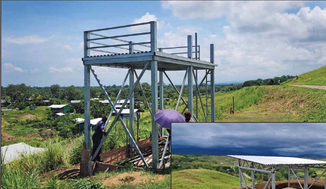
Water Tower under construction
