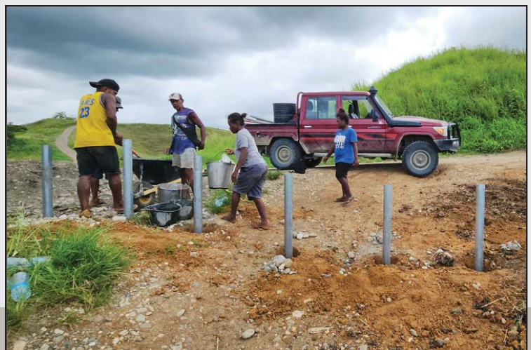
Closure of illegal shortcut road
