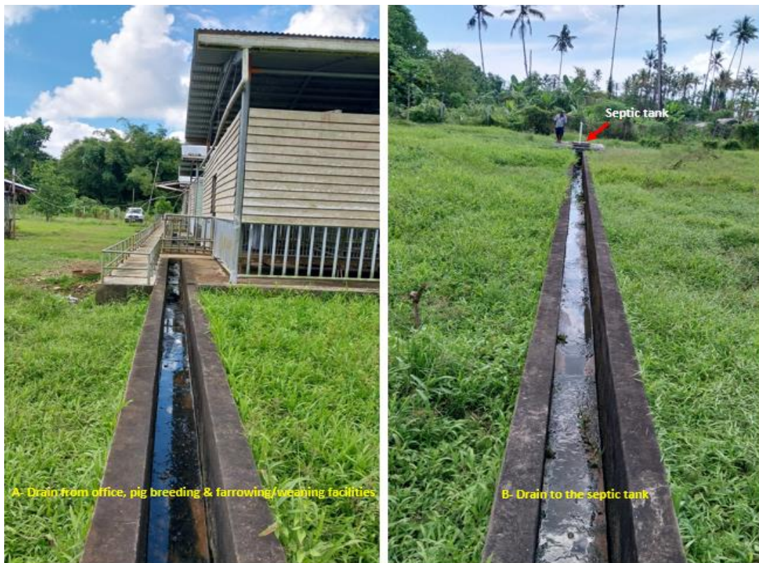
Figure 8: Wastewater management system
