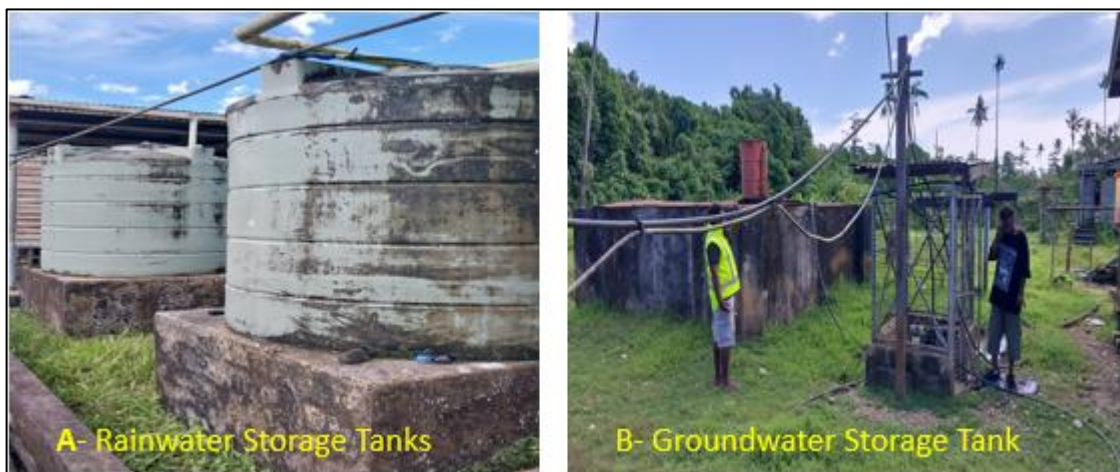
Figure 7: Water Storage facility- A- 2 x 5000 L rota tanks that store rainwater; B- Concrete tank and borehole pump for storage and uptake of groundwater.
