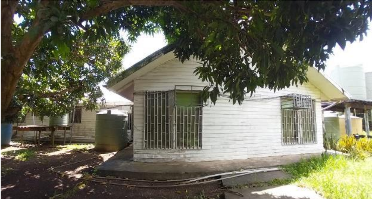
PLATE 8: BACK VIEW OF THE RESEARCH HQ OFFICE
