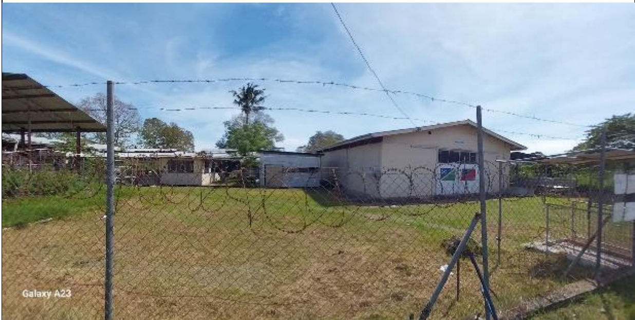
Fig 2: Existing infrastructure of the Slaughter facility
