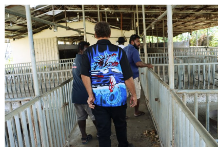
SIART team inspected the KG VI pig breeding facility, slaughter facility, and biogas digester now dysfunctional.
