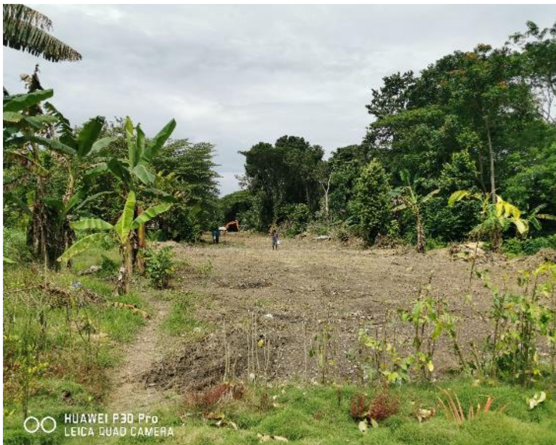
Clearing works at the site
