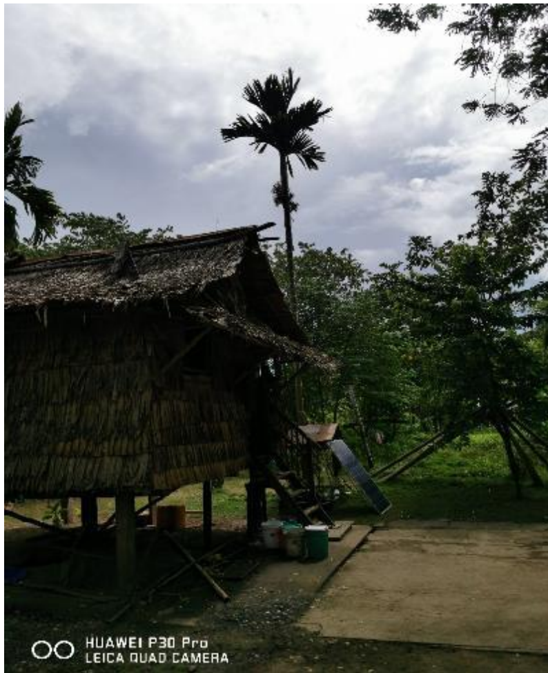
Typical settlers' houses built on remnant concrete slab of former TFES site
