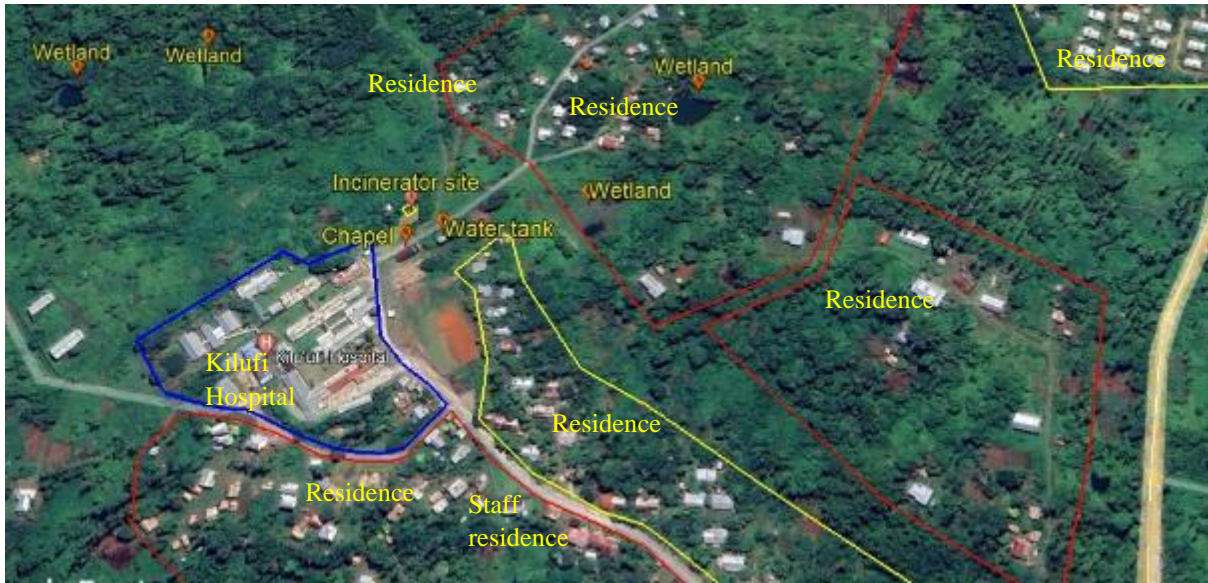
Figure 2.2 Kilufi hospital incinerator site and surrounding area
