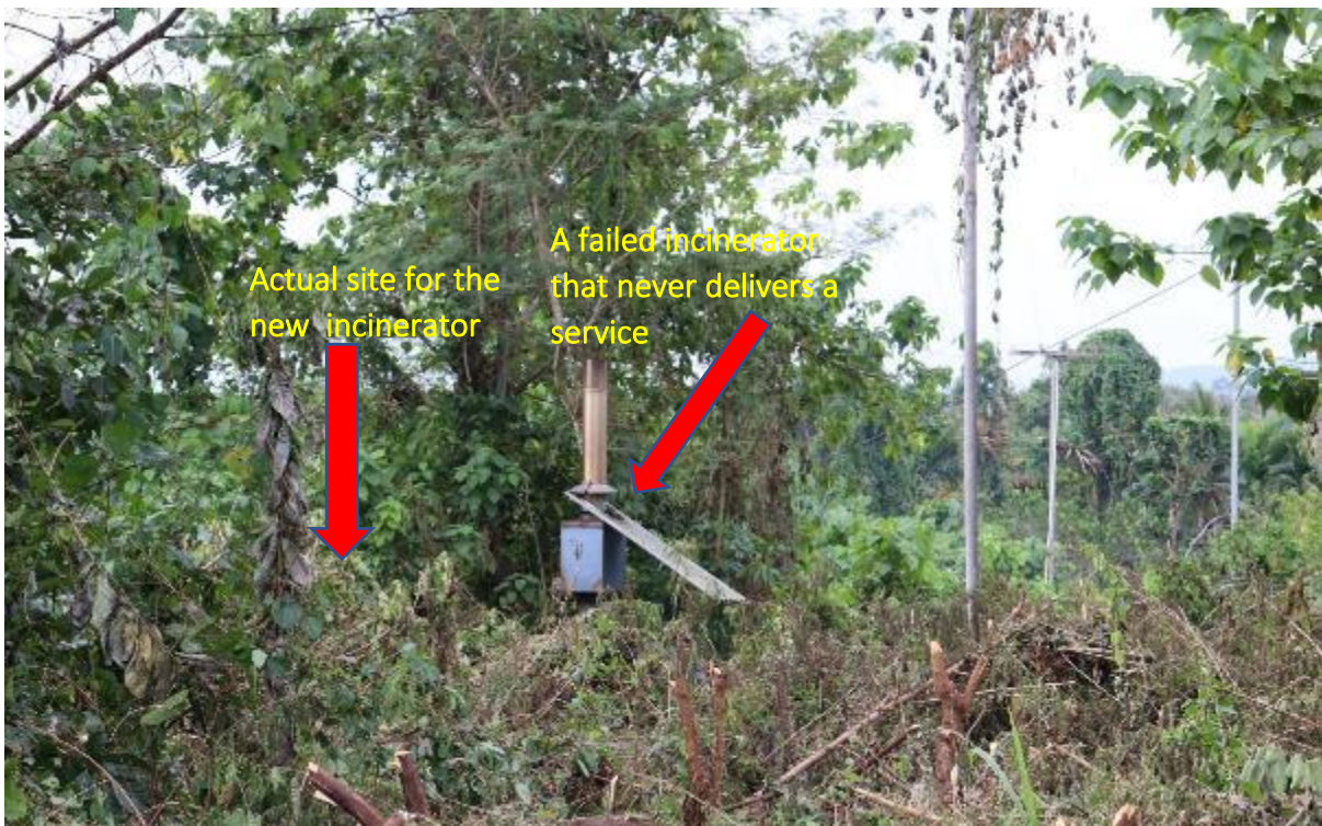
Figure 1.3 Proposed incinerator site photo partially cleared by hospital staff as part of regular hospital compound cleaning.
