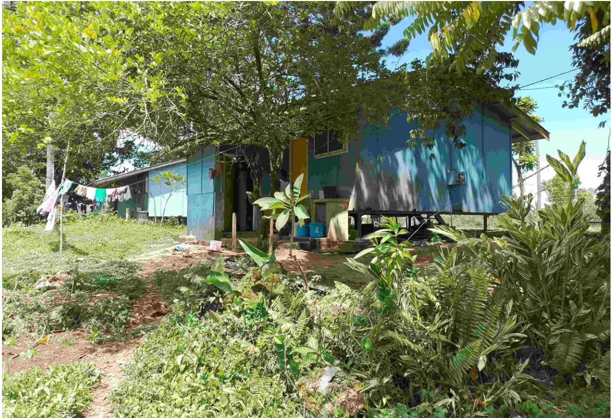
Figure 3.6 Nearby staff houses to the incinerator site
