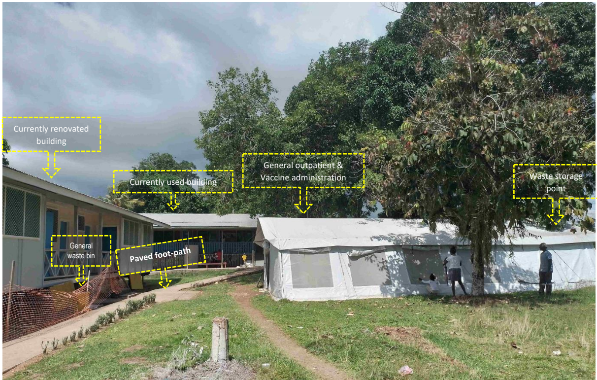
Figure 3.8. Noro clinic compound showing waste storage locations, buildings and access
