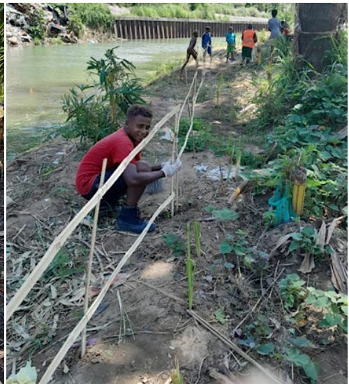
Vetiver grass planting, bamboo replanting, and fencing installation on the riverbank
