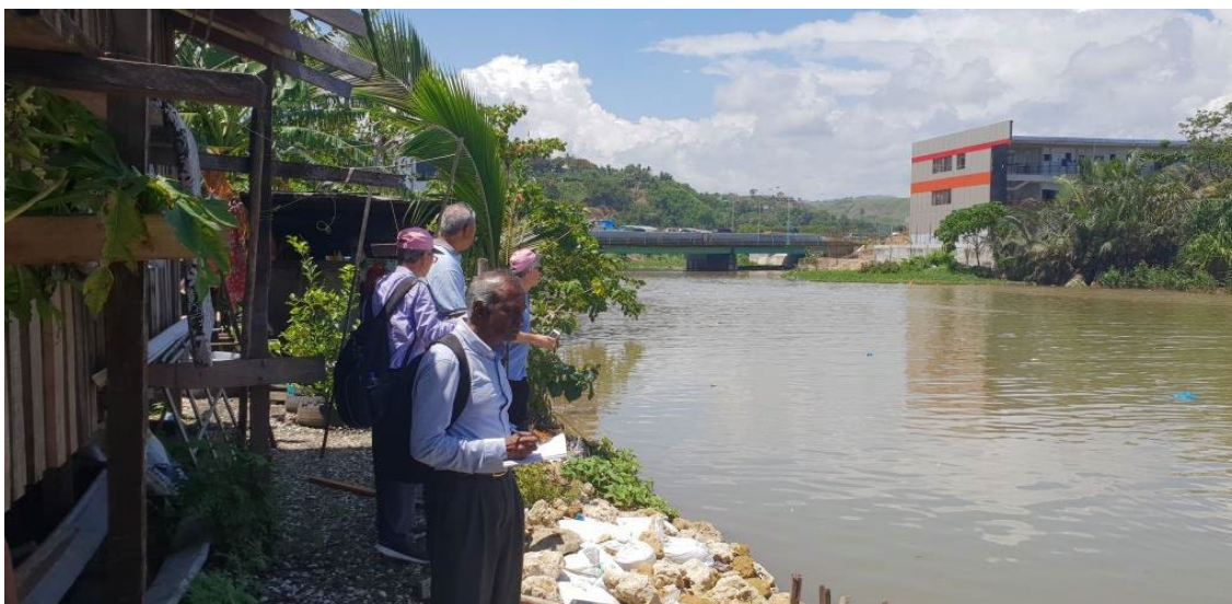
Site visit: RMIT engineers assessing riverbank erosion (Ontong Java settlement).
