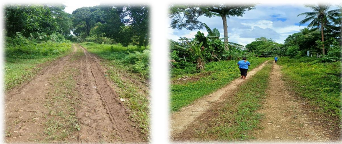
Figure 15: Unsealed access route linking Gizo Township to planned 70-hectare expansion area; subject to major sealing works
