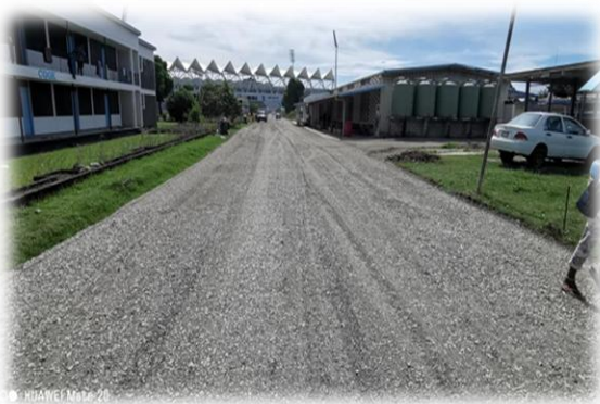
KGVI School road sealing works – SPG related
