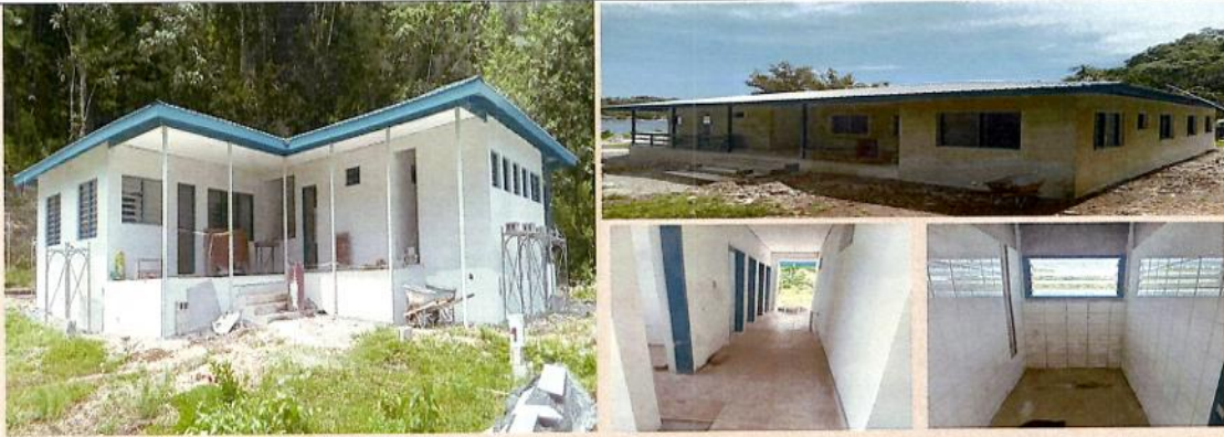
Above captions: Makaa Police Station in 90% completion stage, the photo was taken in February 2024. The Police Station was built by JF Construction, despite many challenges encountered they managed to reach such stage and it was within the project timeframe.
