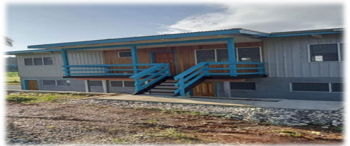
Photo: Malaita Provinc- Aligegeo phase 01 Grandstand project completed and handover in July 2023(MHA)
