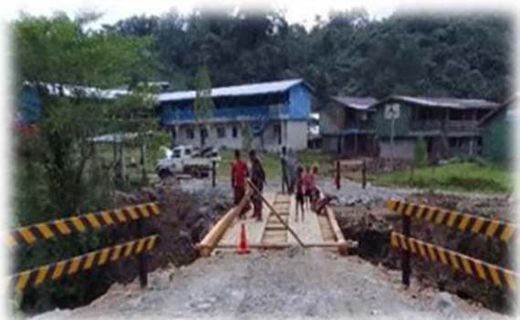
Complete log bridge at Kwaiafa
