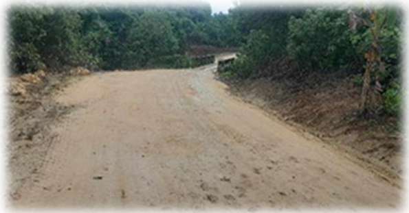
Work in progress on the North road from Dala to Afufu
