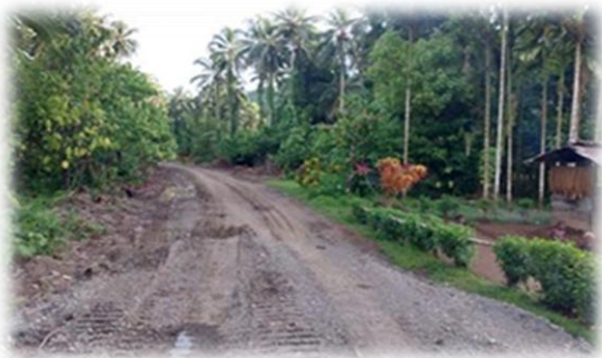
Work in progress on the Marasa Mbabanakira road
