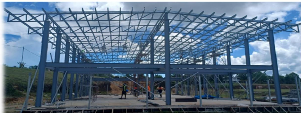
Steel frames and rafters ready in preparation for roofing.
