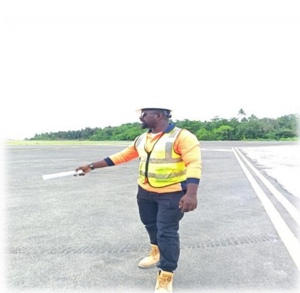
Figure 6: Lata Airport runway upgrade project
