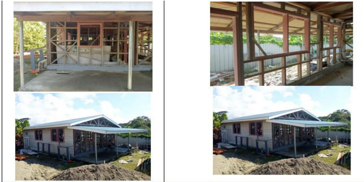
Photo: Rafters, purlins, roofing sheets to the Chief justice quarter (National Judiciary)
