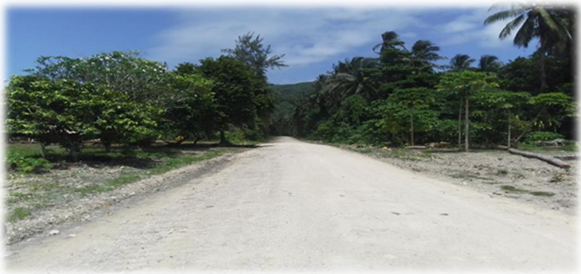
Rehabilitation of Ulawa ring road
