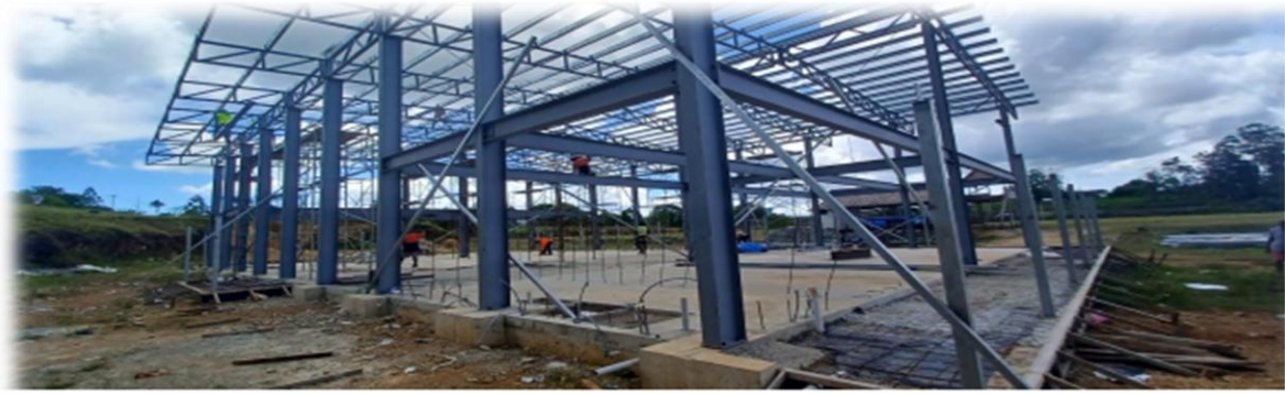
Steel HBM's and Rafters done
