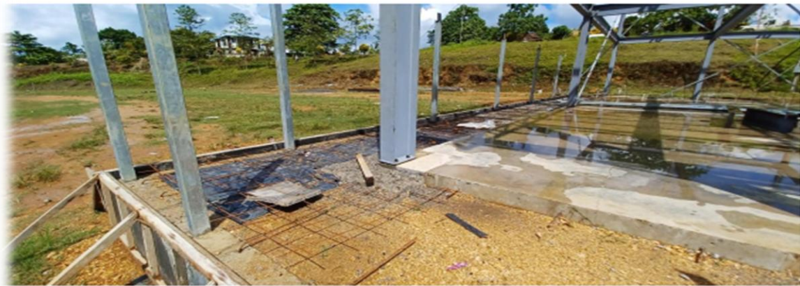
Ground floor concrete basement in progress
