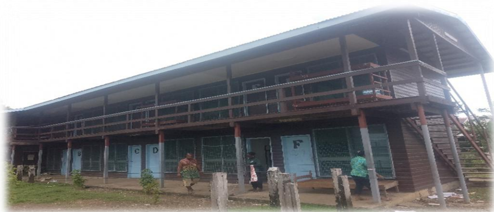
Figure 13: Newly Completed Double-Storey Girls’ Dormitory – Waimapuru NSS
